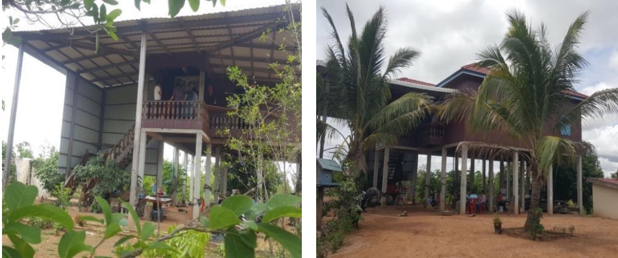
Figure 4: Condition of Existing Homestays in Decho Village
